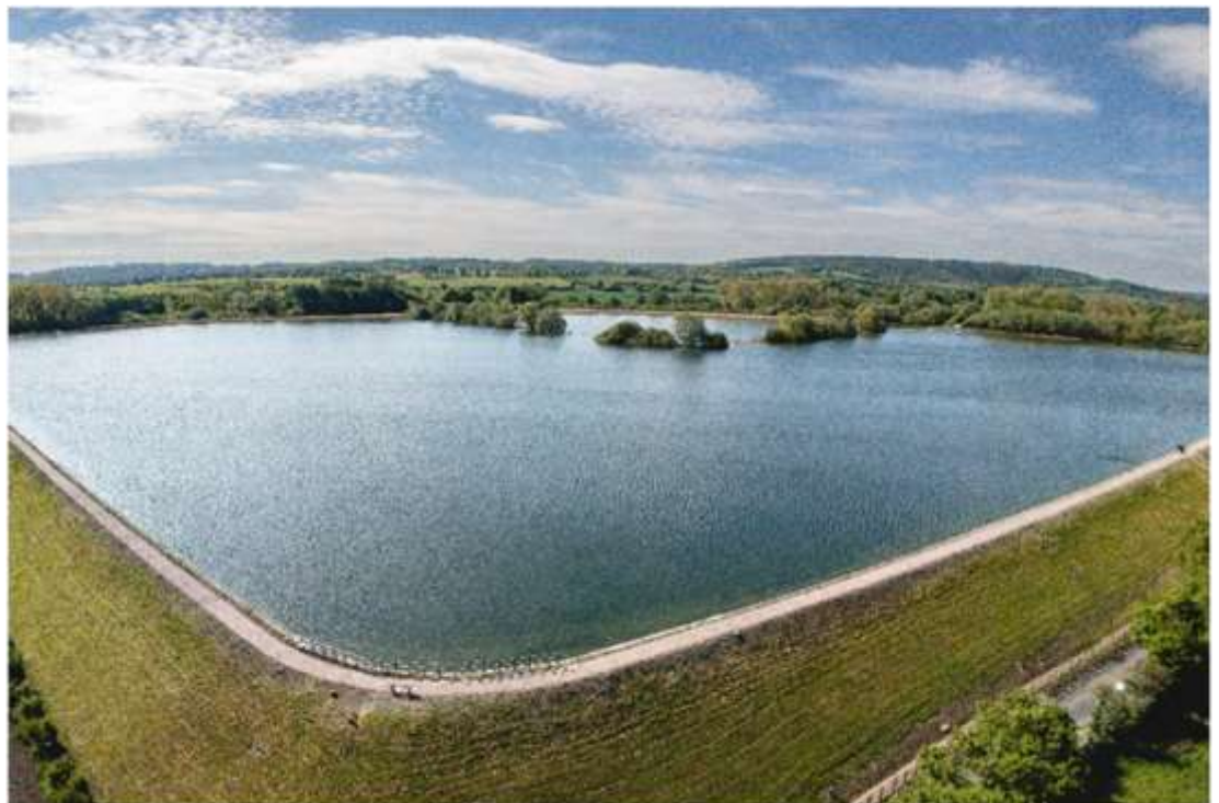
An unusual view of the completed reservoir works
